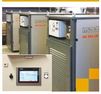
55 kW AG gas compressors used in an installation for an ammonia-based system for removal of CO<sup>2</sup> in Biogas.
